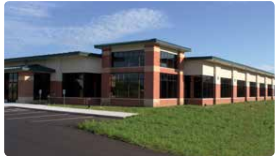
Darley Pump Plant in Chippewa Falls, Wisconsin
